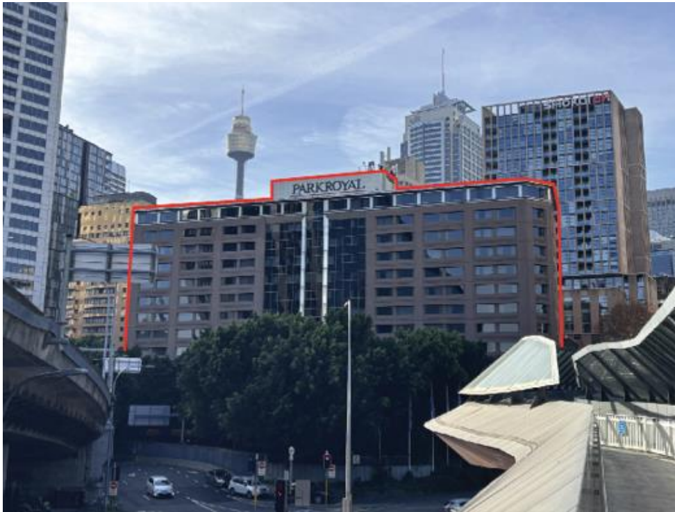
Figure 2: 150 Day Street, western facade fronting Day Street and Cross City Tunnel Harbour Street exit, outlined in red
